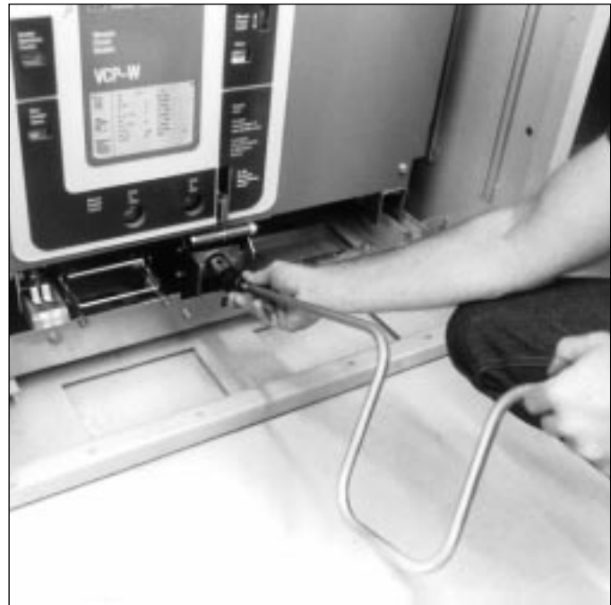
Figure 4-6 Engaging Levering-In Crank
