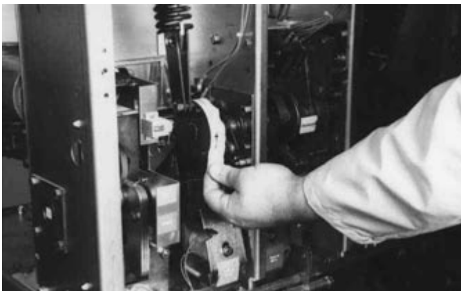
Figure 6-16 Remove Marked Masking Tape from Cam
