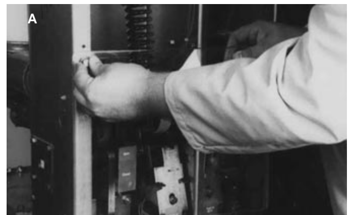
Figure 6-9 Attaching CloSure™ Test Tool at Hole “A”
